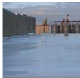
2. Prime surface with Tack Coat™.
