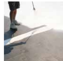
4. Seal entire roof with Rapid Roof III® Top Coat or Equinox® Top Coat.
