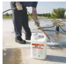
1. Power wash and clean with Wac™ II Roof Cleaner.
