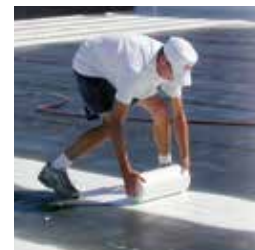
3. Reinforce seams with Spunflex™ embedded in Rapid Roof III® Base Coat or Equinox® Base Coat.
