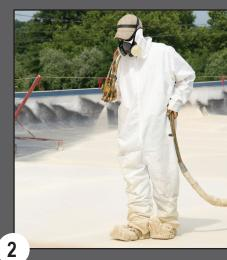
Apply SPF with a minimum thickness of one inch.
