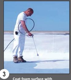
Coat foam surface with appropriate Conklin coating.
